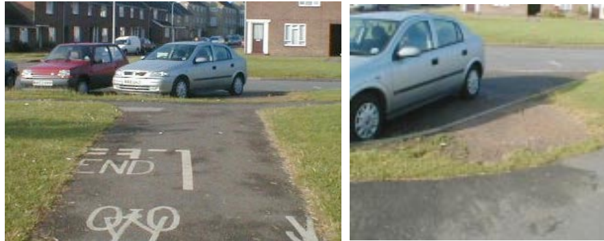
Laurence Avenue. Path ends in a parking bay!
