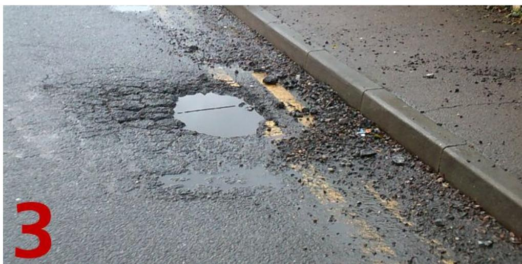
Photo 1 faces West. It shows a rapidly expanding pothole and large sections of crazing between the pink lines. Photo 2 from the same position faces east showing incipient potholes. Photo 3 shows detail of the pothole. From the surrounding debris and state of the adjacent surface it is clear that this is growing quickly.
